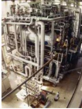
Figure 1. Experimental boiler installation at KEMA.
