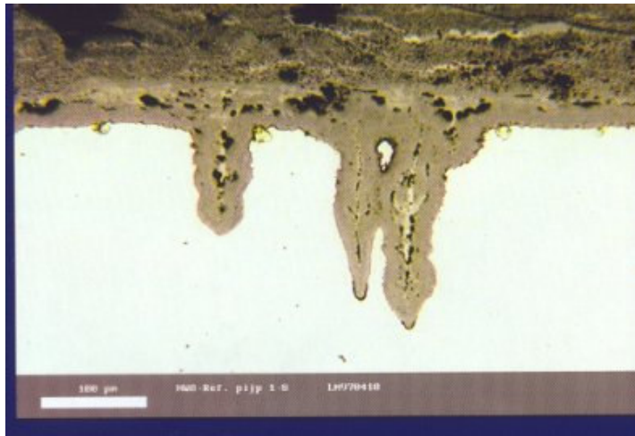
Figure 5 Typical Alligator Skin Cracks in one of the tubes at the rear water wall
