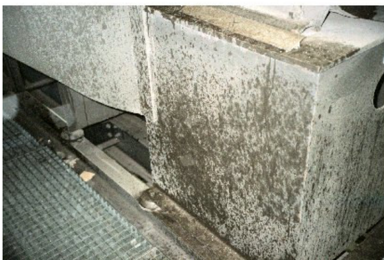
Figure 2 Corroded ventilator
